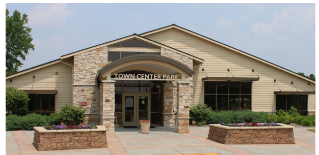
Town Center Park (pictured above) features nearly 24 acres of open space, a playground and a 4,600 square foot community building. It is one of eight parks maintained by Public Works staff.
